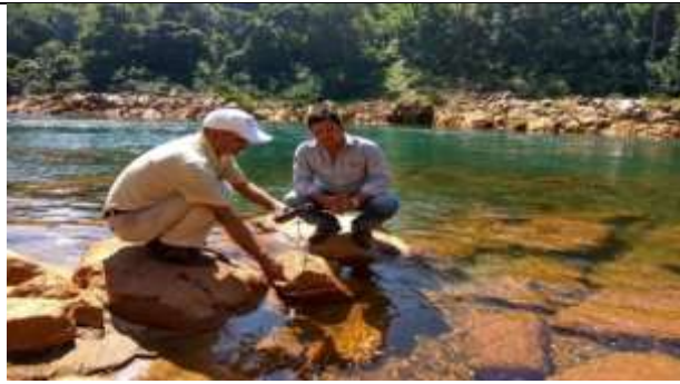
PHOTO 2 : Dam axis, 2.5 km U/S, L/B
